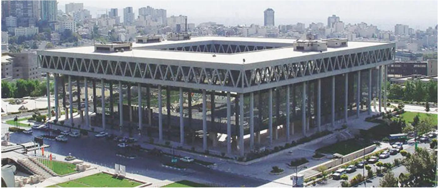
IRIB's headquarters in Tehran
